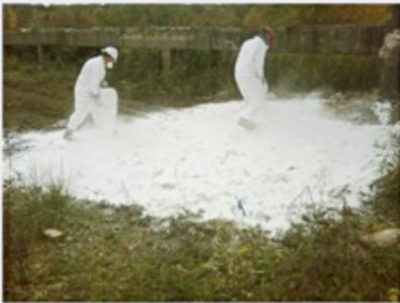
MuniRem ® is directly tilled into the soil for treatment
