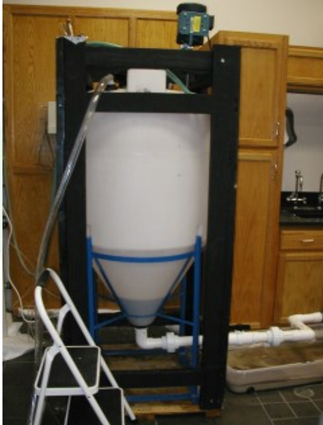
Main Treatment Tank Reactor
